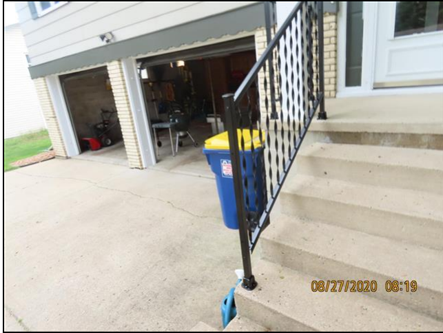
2.0 Item 1(Picture) loose
