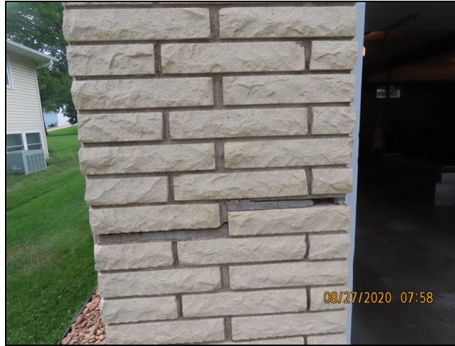
2.13 Item 1(Picture) front left corner of home (garage wall)
