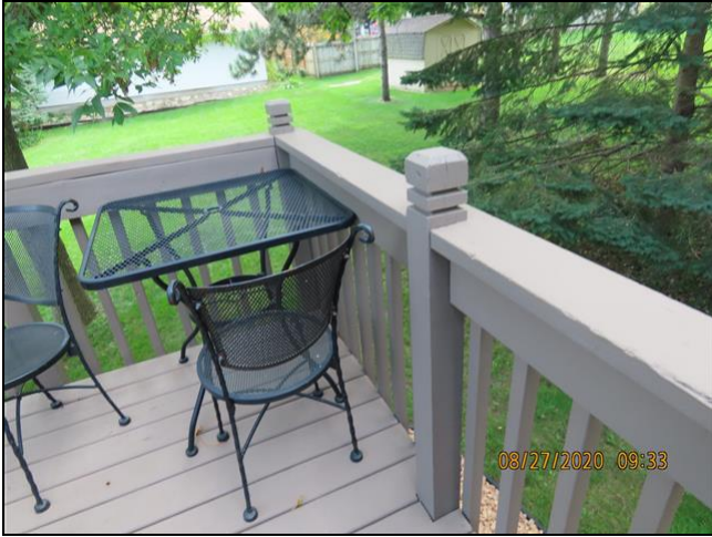
2.7 Item 4(Picture) loose
