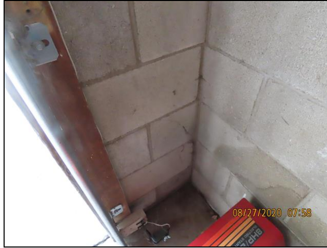
3.1 Item 1(Picture) front left corner of home (garage wall, interior)
