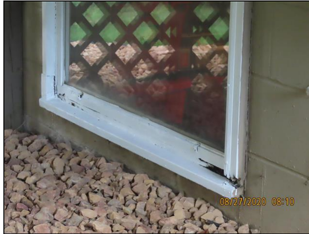
2.4 Item 1(Picture) rear of home, under deck
