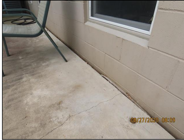
2.5 Item 3(Picture) rear of home
