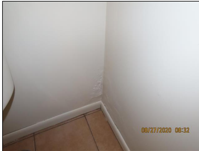
5.4 Item 1(Picture) basement bathroom wall (localized area)
