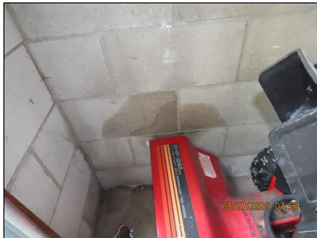
3.2 Item 2(Picture) front left corner of home (garage wall, interior)
