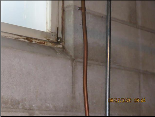
4.7 Item 1(Picture) basement laundry room
